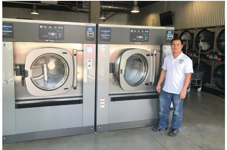
National Laundry & Dry Cleaning, owner Phong Duong added two 90-pound capacity washers to an already robust equipment lineup increasing profit potential without a complete equipment overhaul.
