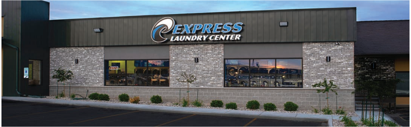
Green Bay Express Laundry Center® sits next to Fast-N-Easy Pawn shop. Owned by Steve Dietzen, the businesses are connected by an interior passthrough — encouraging customer crossflow and management ease.
