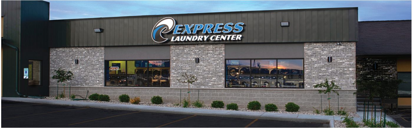
Green Bay Express Laundry Center® sits next to Fast-N-Easy Pawn shop. Owned by Steve Dietzen, the businesses are connected by an interior passthrough — encouraging customer crossflow and management ease.
