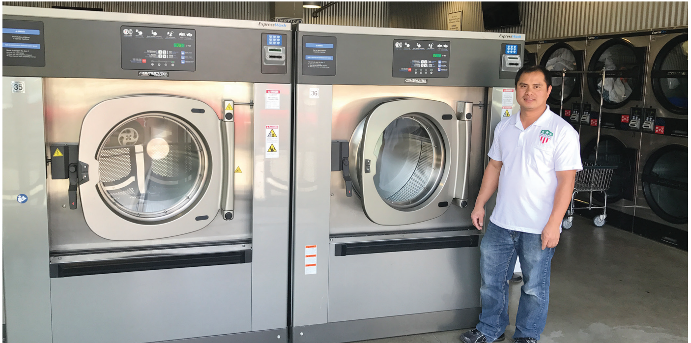
Phong Duong shows off his two 90-pound capacity ExpressWash® washers.
