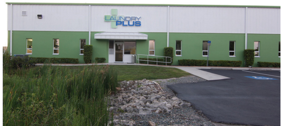
The Laundry Plus operation recently moved to a new plant, where a second GI TBS-50 Continuous Batch Tunnel Washing System was installed. Once that system was fully operational, existing equipment from the old plant was relocated to the new plant, where it was installed, tested and then put into full operation.
