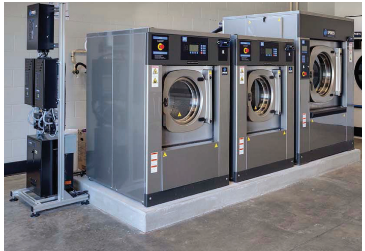
IMG Academy, in Bradenton, Fla., teams two 55- and one 90-pound capacity Sports Laundry Systems washer-extractors with ozone injection, to help prevent the spread of superbugs like MRSA among its student-athletes.
