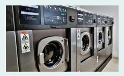
"Unlike hard-mount washers, which must be bolted to concrete foundations, Continental soft-mount washers slide into place without need for bolt-down or grout. This makes it possible to install them in upper-level laundries, like those at The Modern\*."
